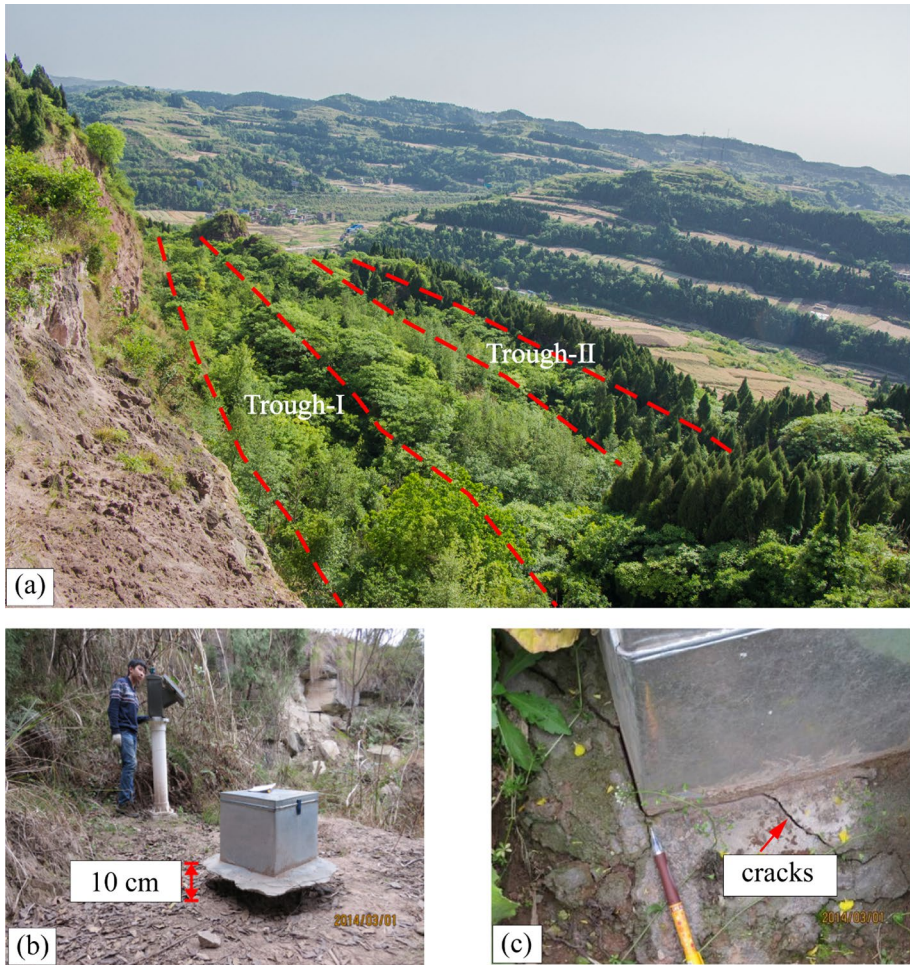
Fig. 3 Historical movements of the Kualiangzi landslide: a two large tension troughs at the rear edge (facing SW20° at the top of Trough-I); b soil settlement observed in the cement pier of a water-level gauge in the middle section of landslide; and c cracking deformation observed in the cement pier of a water-level gauge in the middle section of landslide
