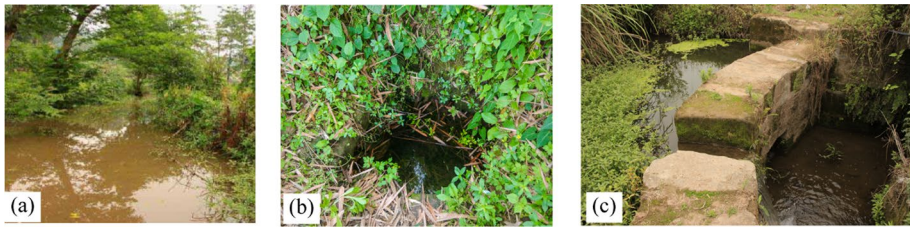
Fig. 5 Recharge and drainage of groundwater in the Kualiangzi landslide: a rainwater storage in the tension trough at the rear edge; b spring drainage at the leading edge; and c channel drainage at the leading edge
