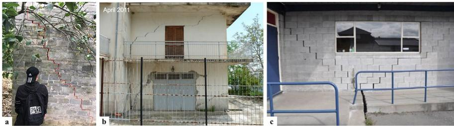
**Fig. 16** The crack pattern of the masonry buildings. **a** The photograph was taken by May 2019, in the Shengjibao landslide. **b** The picture was referred by Antronico et al. (2015). The masonry building located in the Cemetery area, Italy was damaged by the slow-moving landslide. **c** The picture was referred by Somma et al. (2020). The masonry building due to its low tensile strength showed separation of brick–mortar joints
