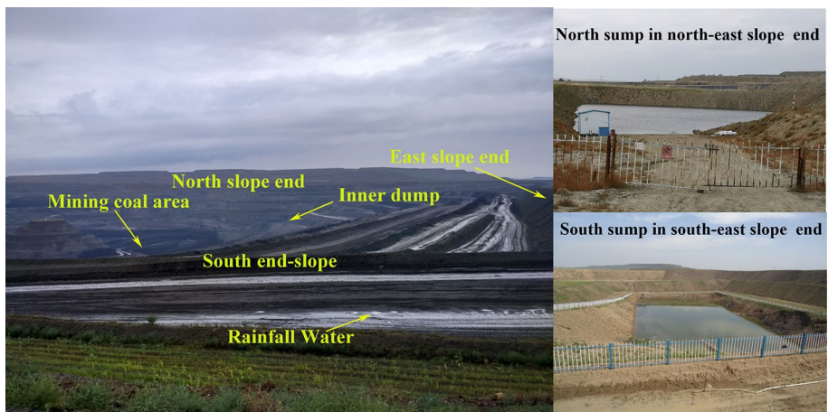
Fig. 3 Field view of the inner dump slope in Shengli open-pit coalmine
