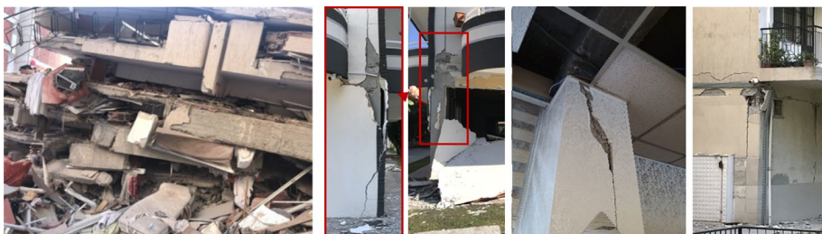
Fig. 14 Strong beam–weak column formation (image by authors and (AFAD 2021; TEC 2018))
