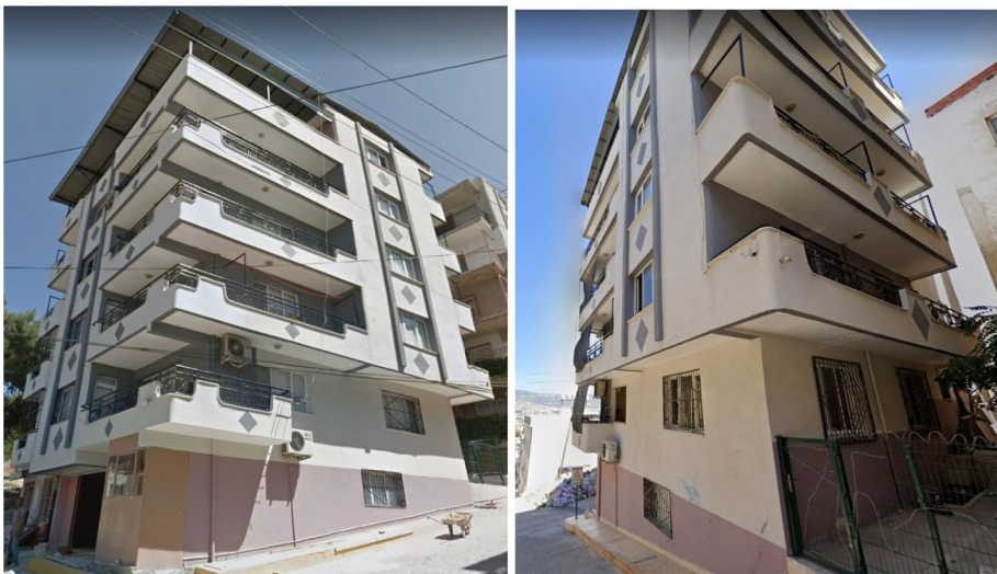
Fig. 21 The current view of the modeled building
