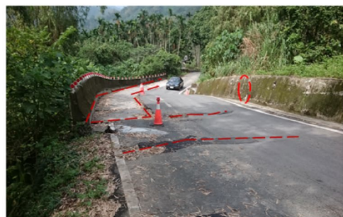
Fig. 23 Cracks in the road surface and lateral translation of retaining wall on side of national route No.135–2 in Taiwan
