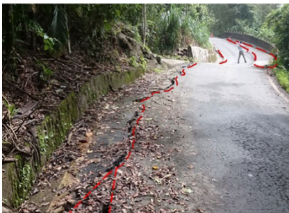
Fig. 23 Cracks in the road surface and lateral translation of retaining wall on side of national route No.135–2 in Taiwan
