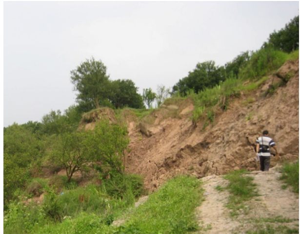
Fig. 19 New landslide on June 7, 2009, at Sai Wan Ba
