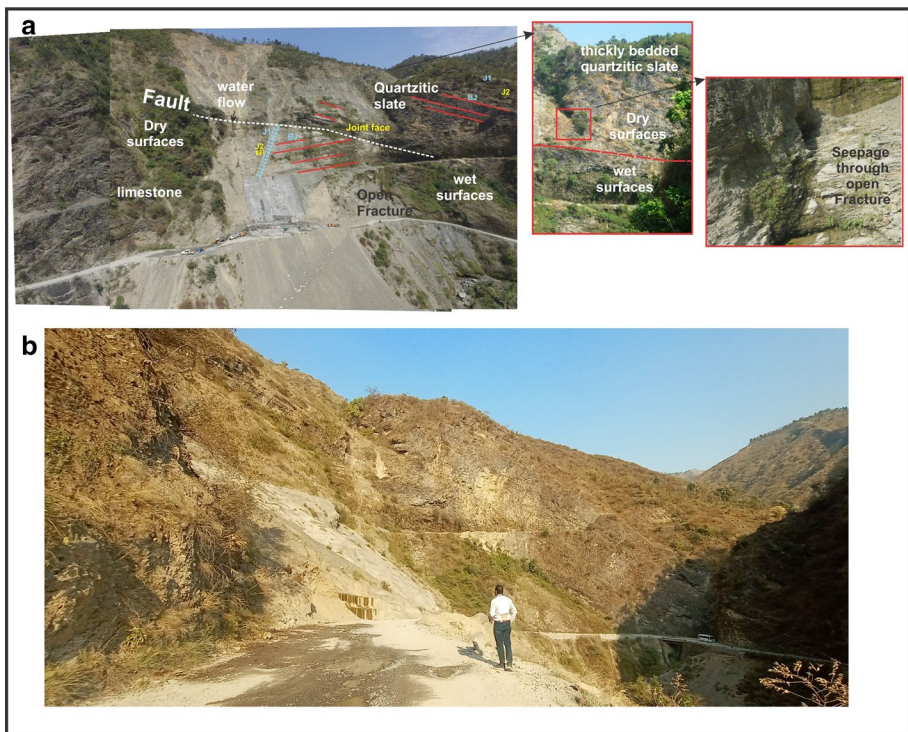
Fig. 12 a Figure depicting the present of fault plane evidenced by changes in dipping direction (marked by red lines). Numerous vertical open fractures developed where seepage is commonly evidences b present scenario of dungale landslide. Note, the road is damaged and showing road subsidence due to clogging of water that seepage out from the landslide site. (Image clicked on April 2021)
