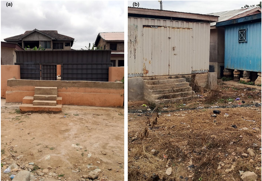
Fig. 12 Ground photographs corresponding to the ground truth points 12 and 16 in Fig. 6, where the height of the boundary walls was measured to indicate the water levels during flooding
