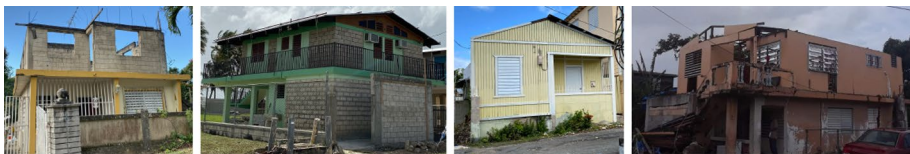
Fig. 2 Photos of Puerto Rican informally constructed houses (Photographs: Polly B. Murray and the authors)
