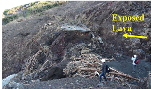
Fig. 7 Eroded surface in the middle of the mountain slope
