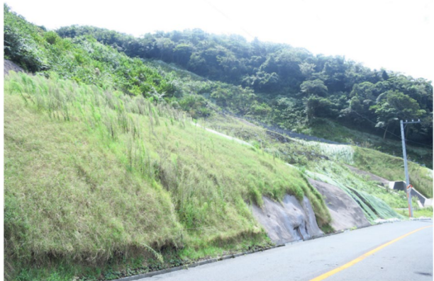
Fig. 38 Intact situation of the monitored slope on September 11, 2018
