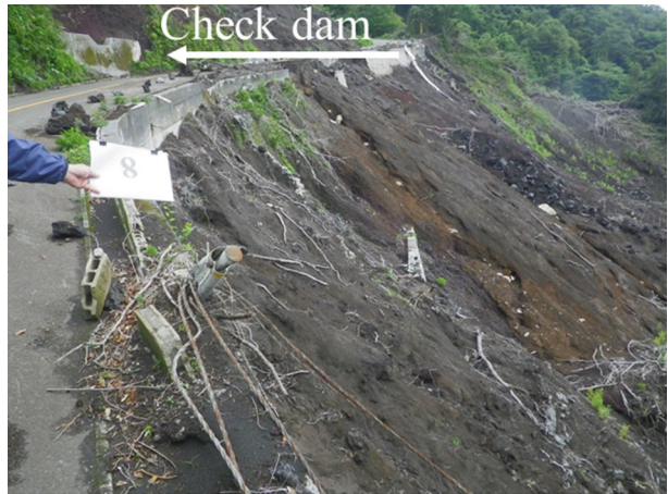
Fig. 20 Post-disaster situation at borehole site No. 8
