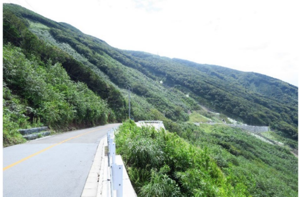
Fig. 37 Intact situation of the failed slope on September 11, 2018 (same site as in Fig. 20)
