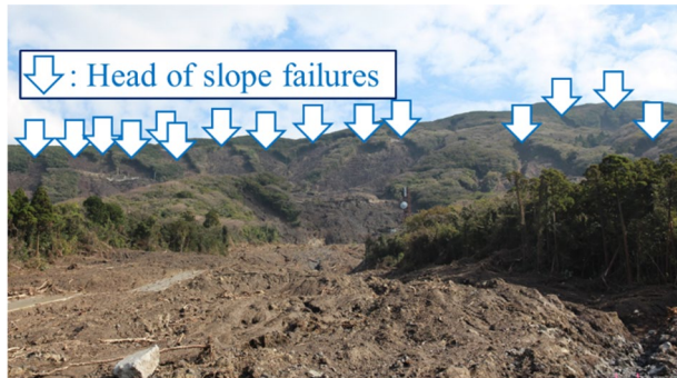
Fig. 5 View of failed slope on the western side of Mihara Yama Volcano
