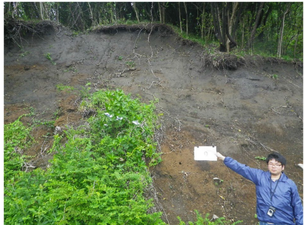
Fig. 21 Post-disaster situation at borehole site No. 9
