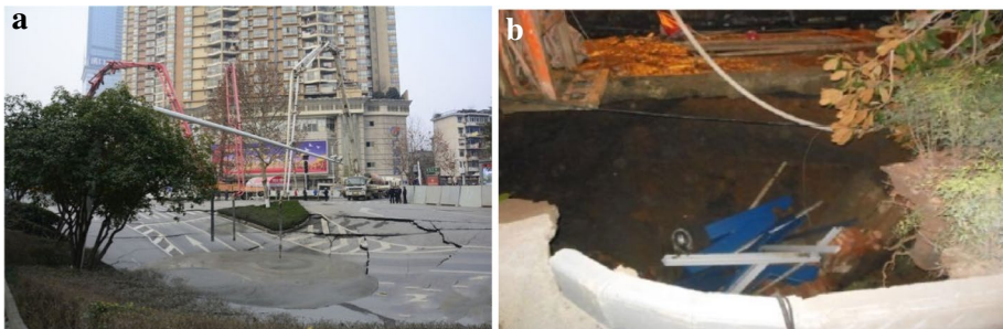
Fig. 7 Photograph of ground collapse induced by shield tunnelling in (a) Wuhan metro line 3 and (b) metro line 6 (Qu 2017)
