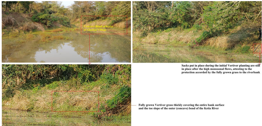
Fig. 7 Views of the right bank of the Ketia (looking downstream), after the Vetiver has fully grown and covered the entire slope surface, with a depicting the difference between the lush Vetiver-enveloped right bank and the sparse untreated left bank and b , c showing the thick coverage and how it envelops each part of the bank surface, including the toe slope. b exemplifies the remarkable stability attained by the right bank, after Vetiver growth, as the sand-filled sacks put in place during the Vetiver planting stage had not been disturbed even during the intervening high monsoonal flows
