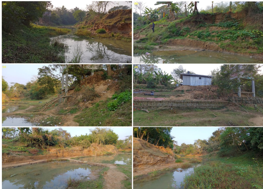
Fig. 8 Views of the unprotected left and right bank of the Ketia River at Gholsai village in January, 2020, with both banks being markedly eroded in the preceding summer monsoonal flows, showing a , c , d the eroded section on the concave right bank upstream of the Vetiver-protected section, even though attempts had been made to protect a portion with just bamboo stakes, but bereft of the Vetiver coverage b rotational bank slumping on the left bank, and e , f sections suffering marked erosion even on the inner left bank, while the opposite Vetiver-protect right bank shows much more stability
