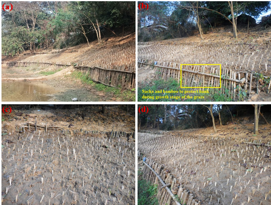
Fig. 5 Recently transplanted Vetiver saplings at Gholsai village ( 22^{\circ} 36' 30'' N, 87^{\circ} 37' 52'' E)—with a , c , and d showing different views, and with b denoting the sand-filled sacks and bamboo cuttings placed on the toe slope and along the bottom of the riverbank in order to protect it while the Vertiver grass grows fully
