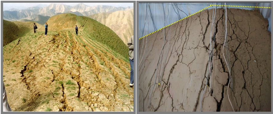
(a) Gedi beam damage of the 1995 Yongdeng Ms5.8 earthquake in Gansu province test
