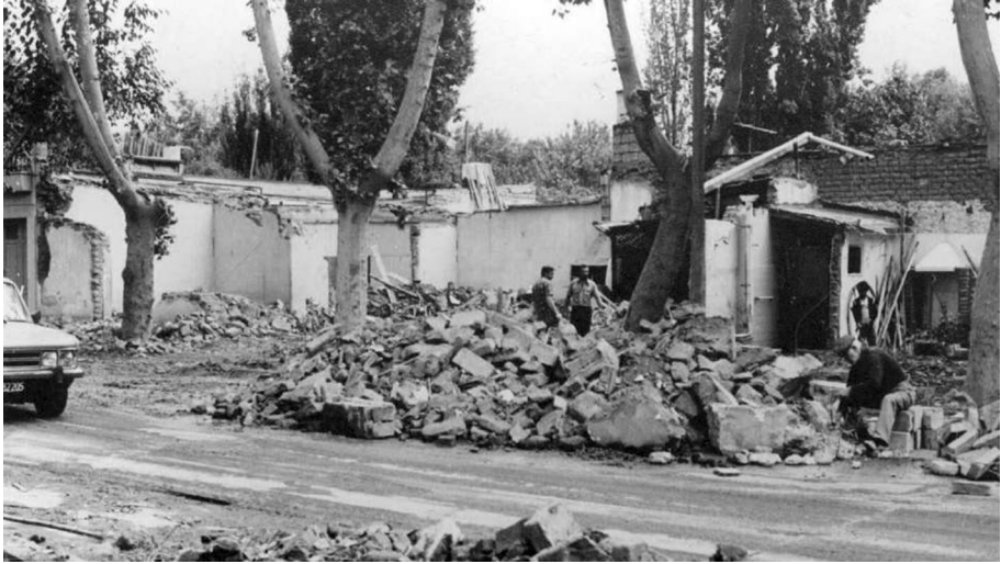
Fig. 4 Totally collapsed houses after the Mendoza ( M_w 5.9) earthquake on 26 January 1985 (Diario Los Andes, Mendoza, Argentina in the 2016 earthquake anniversary edition)
