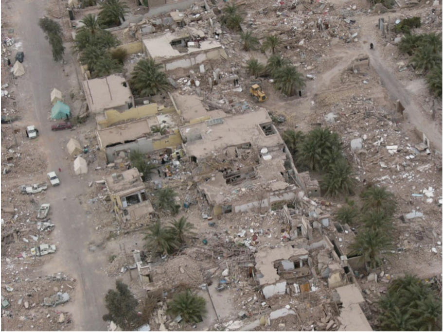
Fig. 21 Severe damages in single story and two-story adobe buildings in central part of Bam city during the destructive earthquake of 2003
