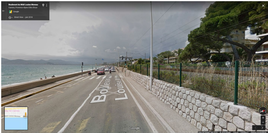
Fig. 9 Coastal road between Mandelieu-la-Napoule and Cannes, bordered by the beach and the railway, view to the WSW (Courtesy of Google Map Inc.)
