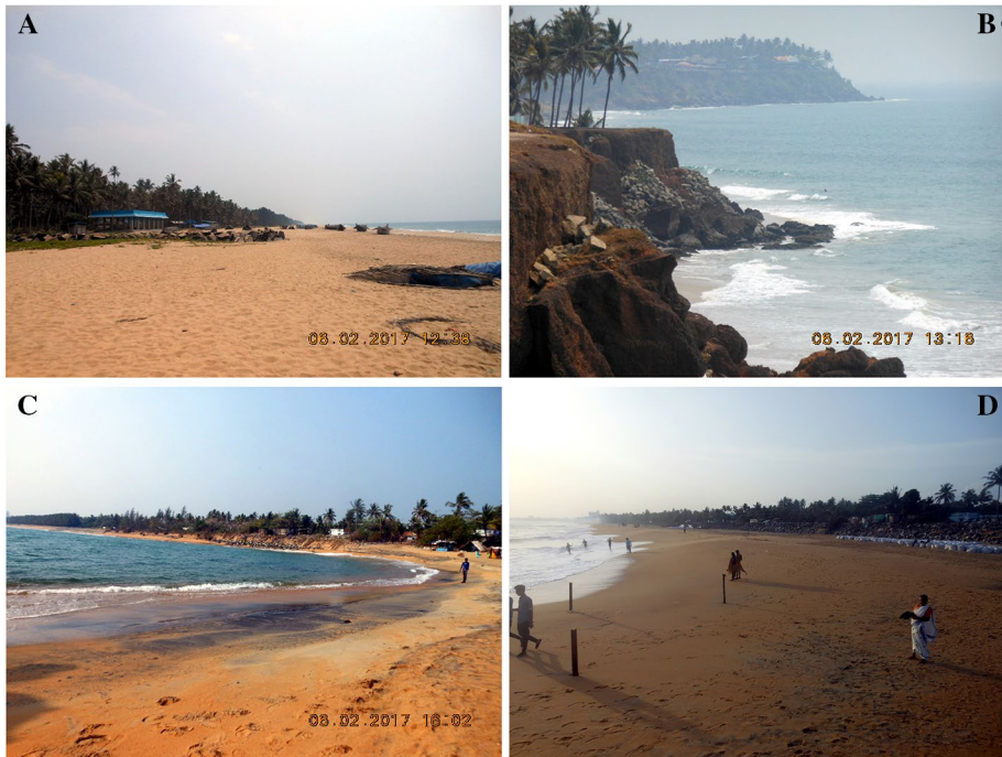
Plate 2 a Rathikkal location where groins were buried in sand. b Slumping of lateritic cliff at Varkala. c Field photograph showing depletion of sand towards the north of broken vessel during pre-monsoon (Feb 2017) at Eravipuram. d Field photograph showing sand deposition towards the north of broken vessel during monsoon (July 2017) season at Eravipuram
