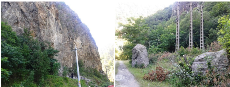
Fig. 12 High-strength slope (SCS 3.51–4.50) and huge fragments of rock detached by sliding (volume = 48 m 3 ) to quarry excavation from Muntele Cărligul Mic (06.VII. 2017)
