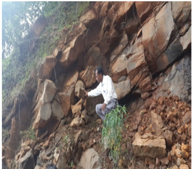
Fig. 2 Landslide due to failure of joints
