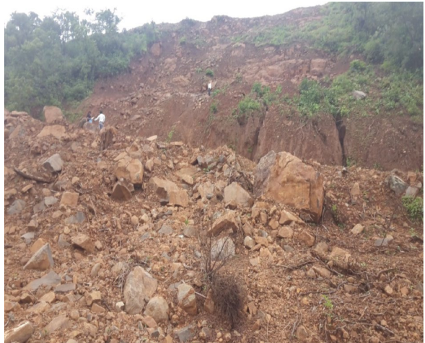
Fig. 1 Landslide due to heavy rainfall
