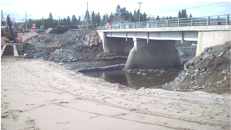
Fig. 5 Pibrac Bridge: for high discharges, the pillar is an obstruction to the flow, increasing the water level upstream. Note the cofferdam installed to limit suspended sediment release
