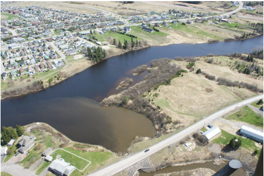
Fig. 9 Suspended sediment inflow from tributary C (km 5.4) (Courtesy of GENIVAR)
