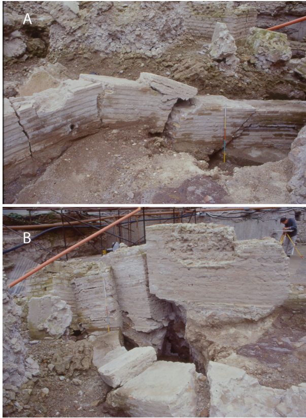
Fig. 6 Villa Medici: a, b remains of the disjunct and displaced walls, at an elevation lower than that of the original surfaces
