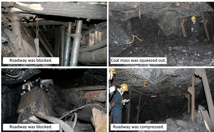
Fig. 1 Serious destruction of mining roadways and machineries induced by the rock burst occurring in a deep underground coal mine
