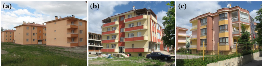
Fig. 11 Examples of RC buildings from Erzincan; a shear wall RC building (RW), b frame RC building (RF), c dual RC building (RH)
