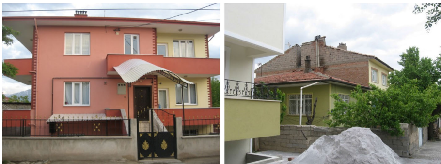
Fig. 12 Examples of masonry buildings from Erzincan with varying material and construction quality
