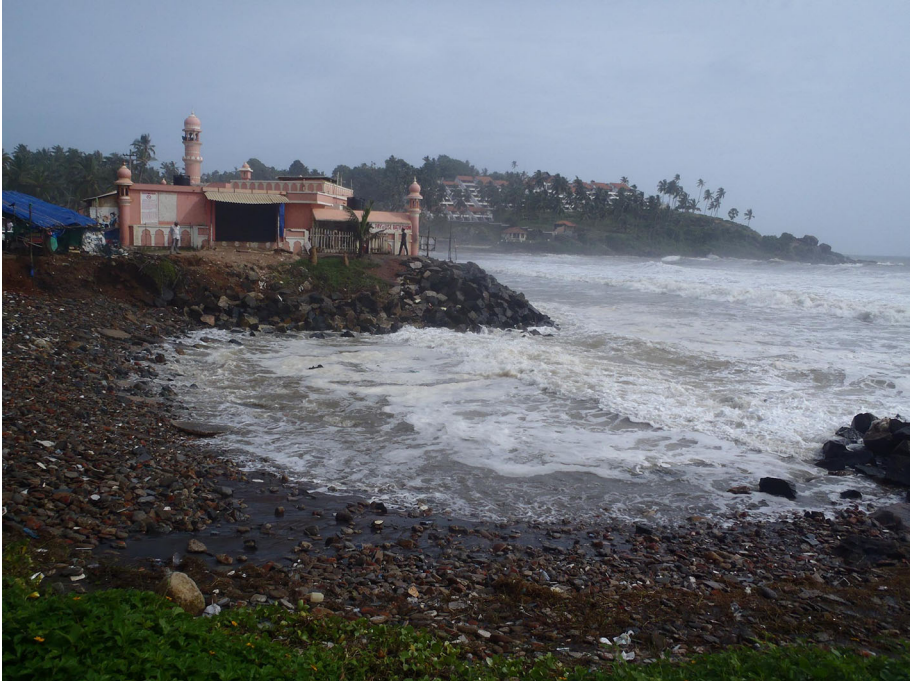
Fig. 15 Impact of building construction on a stable pocket beach at Kovalam
