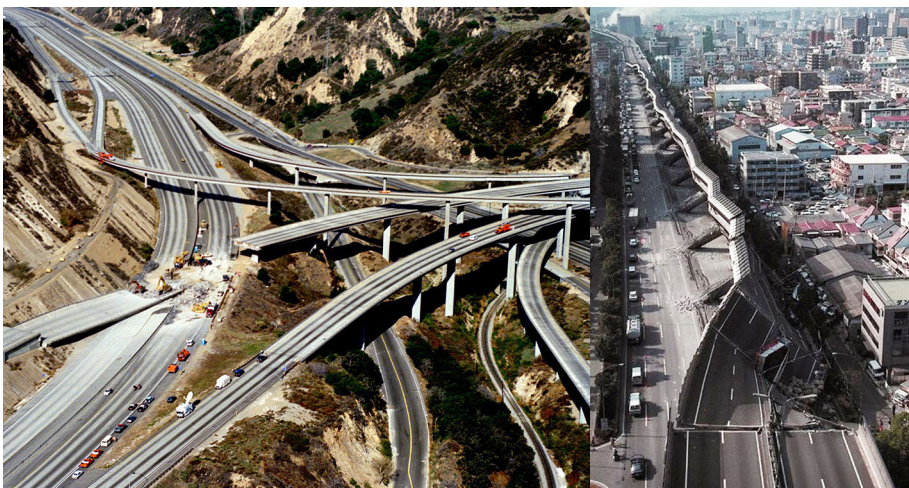
Fig. 1 Photographs of the freeways affected directly by the 1994 Northridge Earthquake (left) and 1995 Great Hanshin Earthquake (right). Sources: Paul Harris/Getty Images and Yozo Fujino
