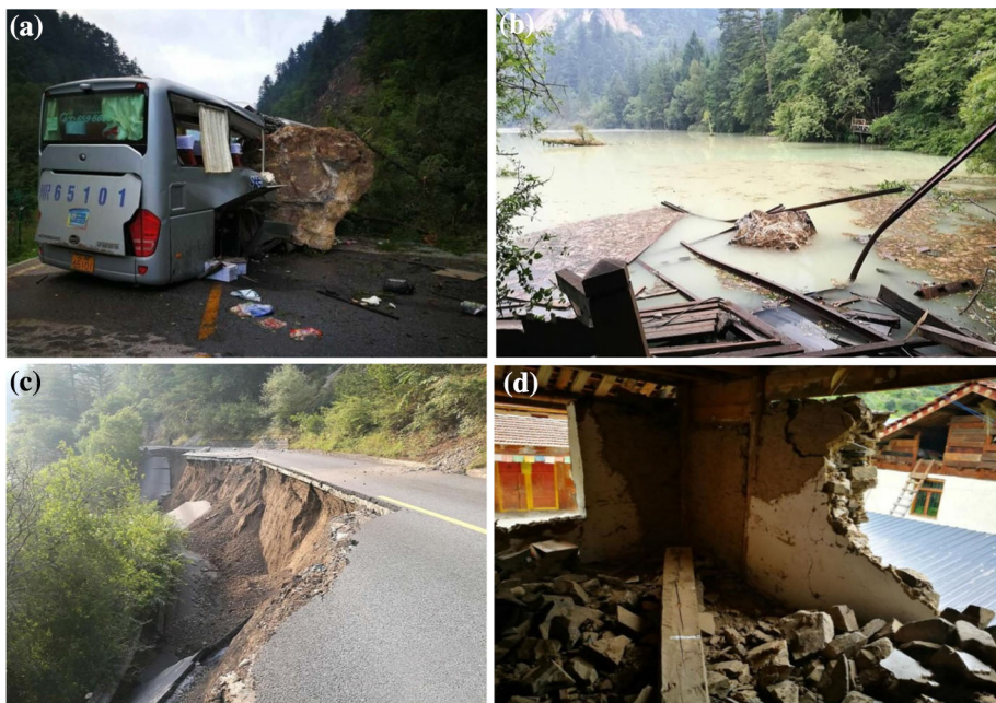
Fig. 4 Maps of damages after Jiuzhaigou earthquake. a Bus damaged by falling rocks; b infrastructure damage in scenic spot; c road collapse; d house damage. Sources: http://www.xinhuanet.com/ , http://www.chinanews.com/ and China Earthquake Administration http://www.cea.gov.cn/
