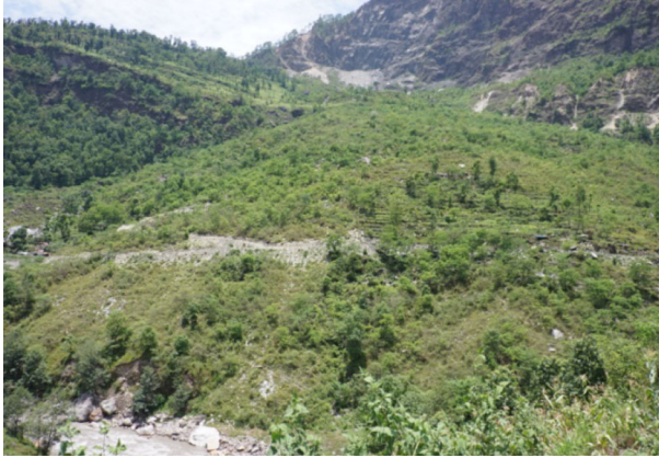
Fig. 26 Large developed ancient landslide body to the west of the main trench (facing west)
