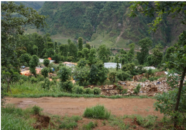
Fig. 24 A completely collapsed stone masonry structure at the school gate (facing west)
