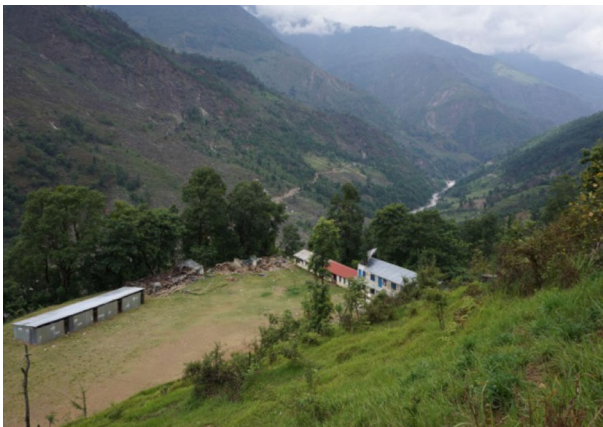
Fig. 25 School houses were severely damaged (facing west)
