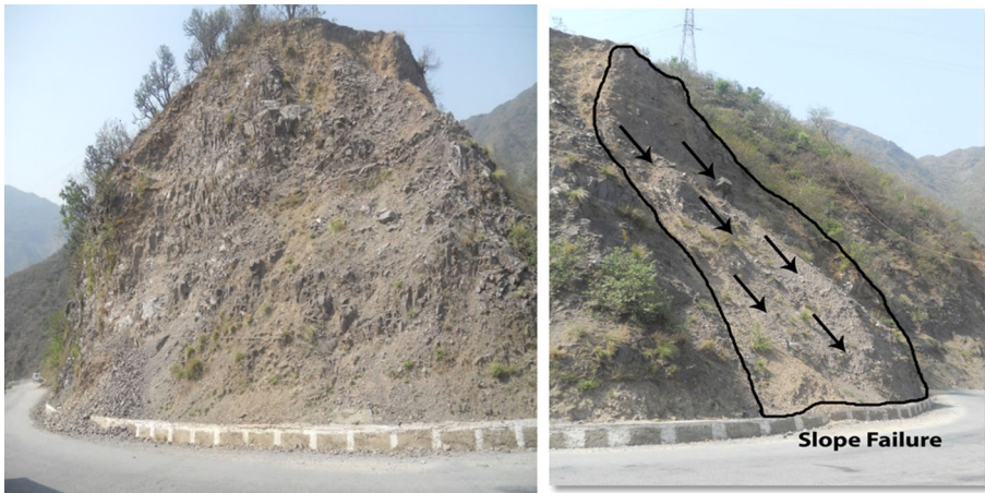
Fig. 3 Investigated slope along NH-58, near Saknidhar, Uttarakhand
