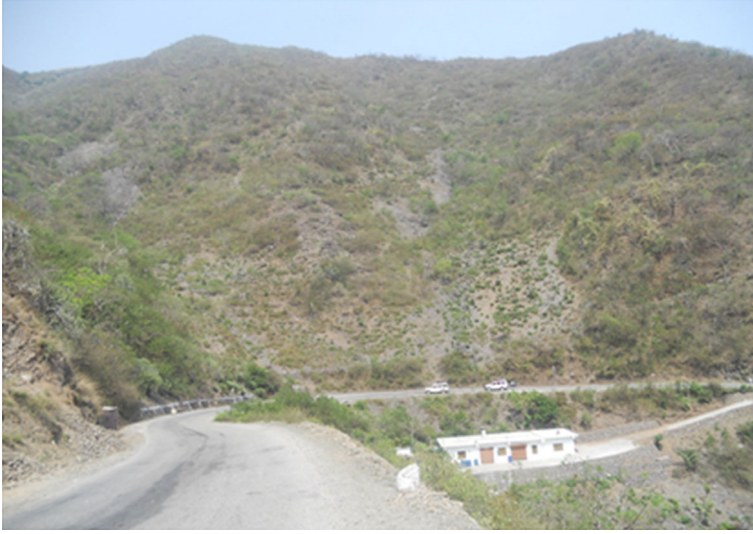
Fig. 2 An overview of the cliffs, hills and roads in Uttarakhand along NH-58
