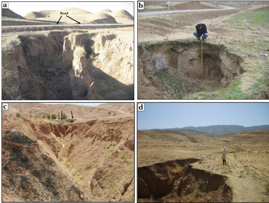
Fig. 2 Field photographs of some gullies occurred in the study area; the gullies are hazardous to anthropogenic infrastructures such as roads and buildings (a–c), and agricultural lands (d)
