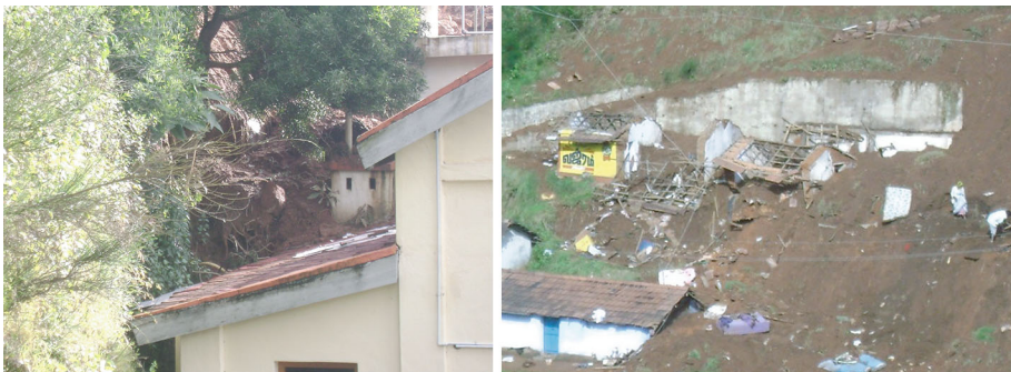
Fig. 4 Damaged buildings due to 2009 November landslides
