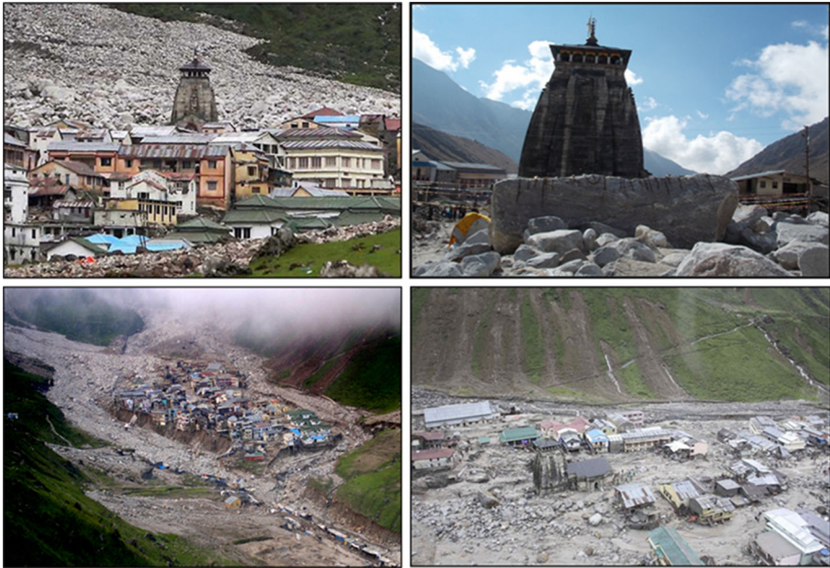
Fig. 3 Photographs showing the impact of flash flood surrounding the Shri Kedarnath Temple
