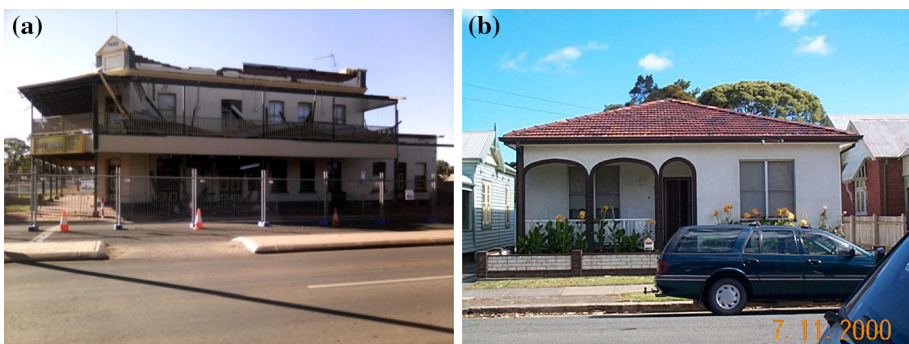
Fig. 4 Example of unreinforced masonry (URM) structures. a An example of pre-1945 brick commercial building. b An example of post-1945 brick residential building
