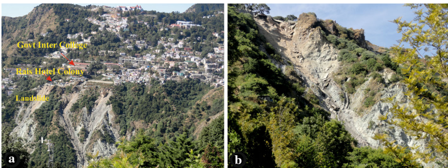
Fig. 8 a Panoramic view of the Rais Hotel colony landslide that has damaged about 20 houses and is endangering the entire Rais Hotel locality including the GIC, b main body of the landslide depicting weathered rocks in landslide zone and is covered with thin veneer of sediments
