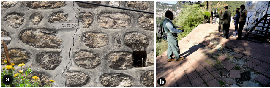
Fig. 6 a Cracks surfaced again and in continuously widening on the retaining wall in a school building that was repaired in 2010 and b tiles of the floor have been uprooted in a zone of about 2 m width and more than 50 m length in the Kailakhan region on the left flank of the Balia Nala
