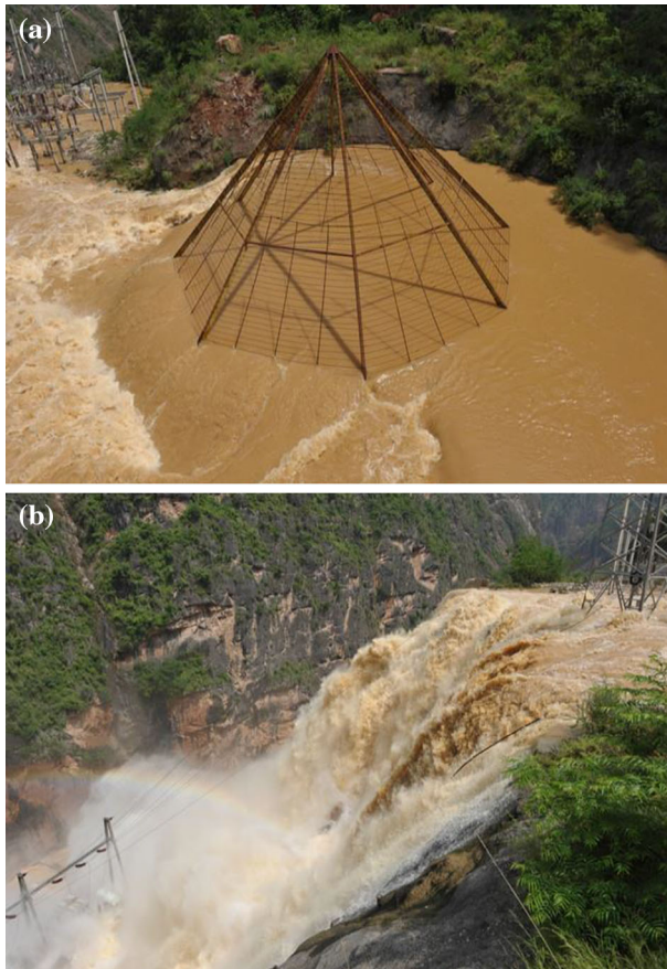
Fig. 5 Overflowing through the surge tank
