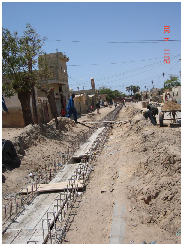
Fig. 3 Construction of new drains and sewerage in Diaminar (Picture: Trond Vedeld 2012)
