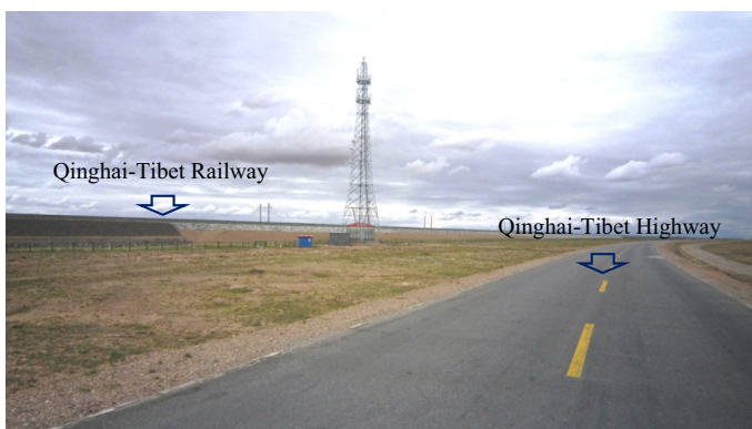
Fig. 1 Example of transportation infrastructure in the Qinghai-Tibet Engineering Corridor
