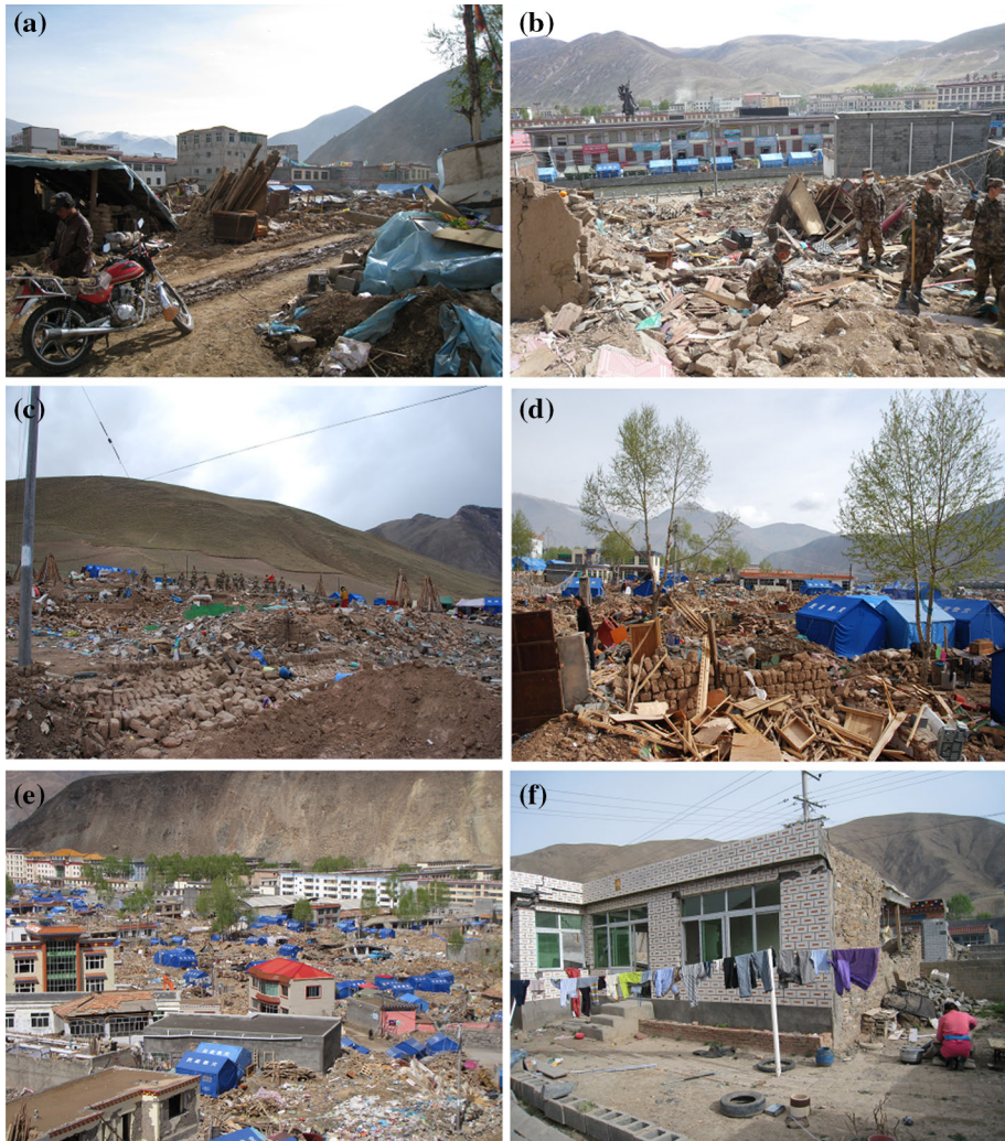
Fig. 5 a Complete destruction of 16 single-story adobe houses with timber roofs near Shengli Road (Part IV), b 12 collapsed adobe houses with timber roofs near Hongwei Road (Part V), c complete destruction of more than 60 adobe houses with timber roofs in Saiyigou Village (Part II), d more than 70 collapsed adobe houses with timber roofs in Shuangyong Lane (Part I), e complete destruction of adobe buildings versus standing of other buildings around North Xihang Road (Part II), f partially collapsed gables and cracked interior walls in a single-story stone house near Qionglong Road (Part V)
