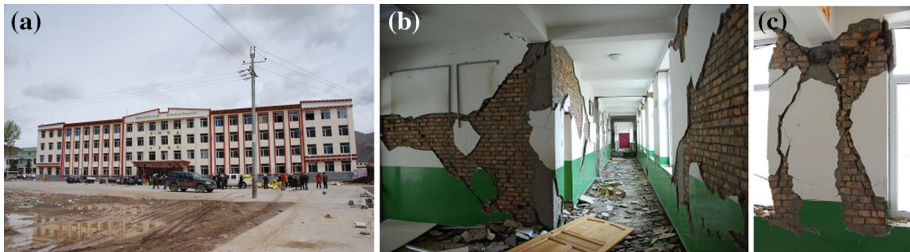
Fig. 17 X-shaped cracks in most bearing walls, and broken columns on the first floor of a four-story masonry building of Yushu First National Middle School that was constructed using cast slabs, columns, and belt courses (Part IV)
