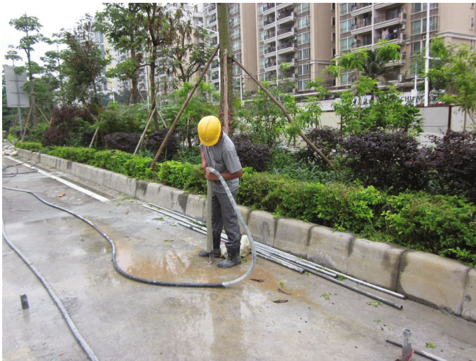
Fig. 6 Slurry grouting into the karst cave
