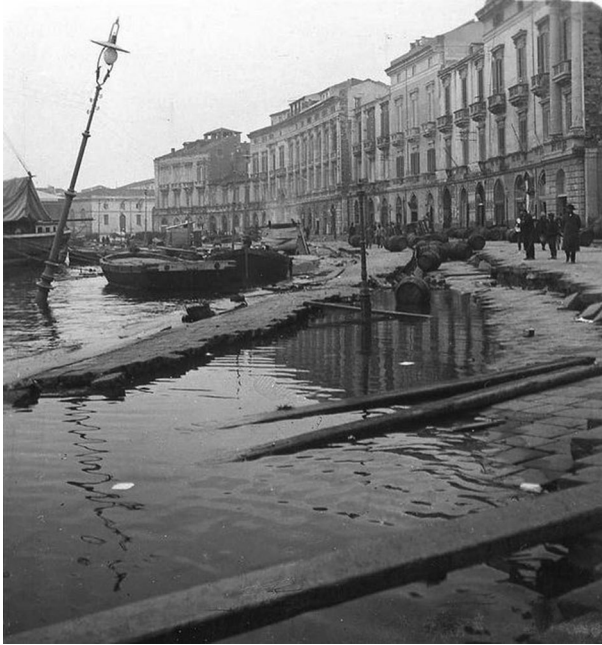
Fig. 17 Messina waterfront before the “Palazzata” was damaged by the combined action of the earthquake and the tsunami. Seismic shaking, liquefaction, and lateral expansion presumably induced the failure of the bearing structure of the wharf (photograph: L. Comerio 1908)
