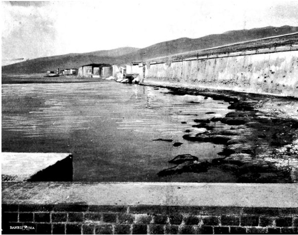
Fig. 25 Don Blasco Bastion resting on panchina type deposits uncovered by the tsunami waves (Franchi 1909). See Fig. 8 for location
