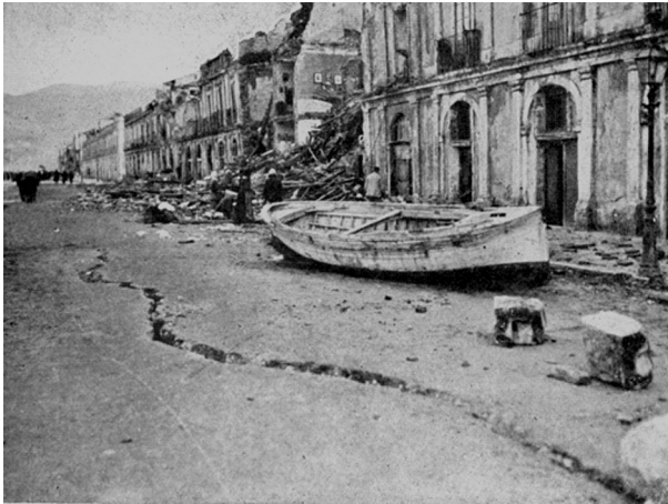
Fig. 20 Ground crack along Marina Street, Reggio Calabria (Baratta 1910)
