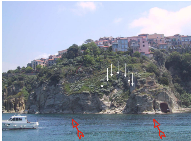
Fig. 6 View of the landslide crown of a wedge failure affecting the Agropoli promontory. Several discontinuities near parallel to the predominant wave direction (represented by the red arrows ) can be also observed
