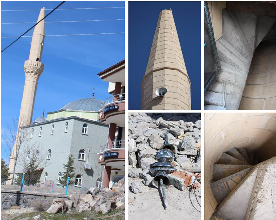
Fig. 2 Slightly damaged minaret at Elmacik Village
