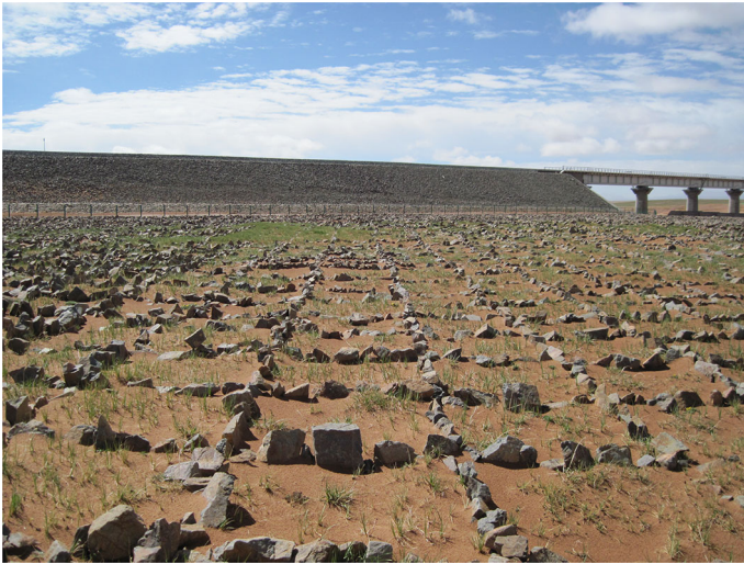
Fig. 13 Grasses in the sand barriers of rocky grid at Honglianghe River section of Qinghai–Tibet Railway (Aug 2014)
