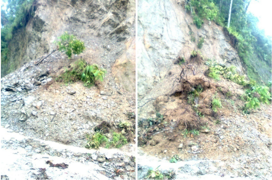
Fig. 3 Landslides of Sirwani village
