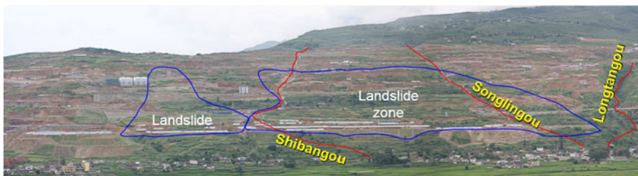
Fig. 1 Panoramic photograph of the new Hanyuan County on the hillock. The blue lines indicate the approximate boundary of the main landslides, and the red lines represent three ditches through the whole resettlement zone
