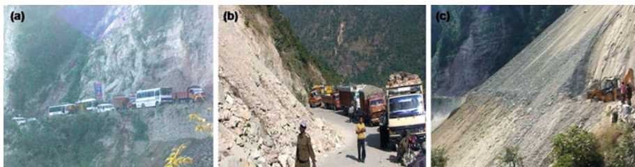
Fig. 5 Vehicles trapped on both sides of NH 58 (a, b), during restoration work (c)
