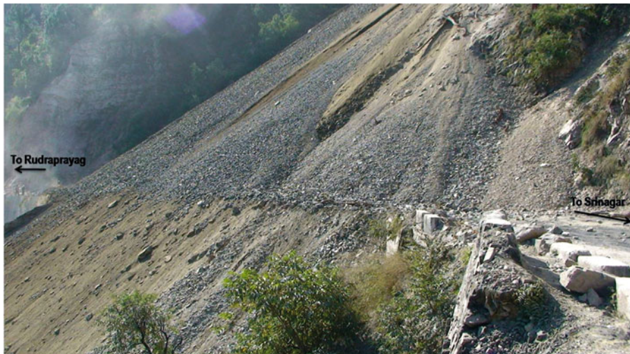
Fig. 4 Blockade of Highway due to large volume of debris generated
