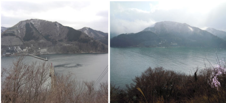
Fig. 7 Breakwater at Onagawa town before ( left ) and after the tsunami. Note that the tsunami completely destroyed the breakwater, with the caissons being scattered by the incoming and outgoing wave
