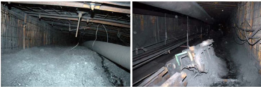
Fig. 16 Gas outburst accident at the No. 10 coal seam in the Haizi Coal Mine
