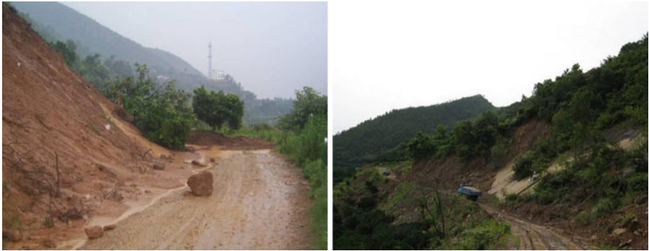
Fig. 3 The scene of landslide collapse along roads on June 30, 2007
