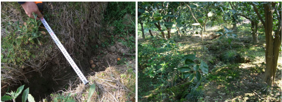
Fig. 4 Landslide fissure in the warning zone
