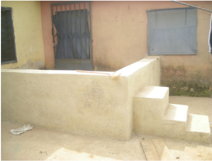
Fig. 8 An individual adaptation to flood by building a wall around the door to a room in a compound house
