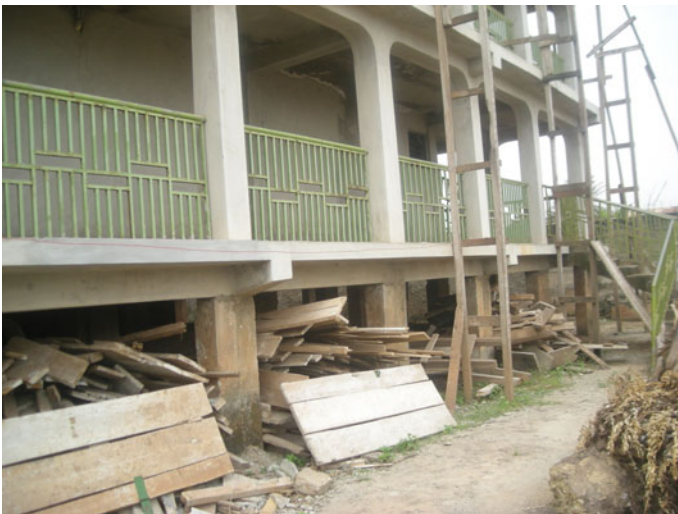
Fig. 11 Adaptation to floods by construction on a house on stilts in a flood-prone suburb in Kumasi
