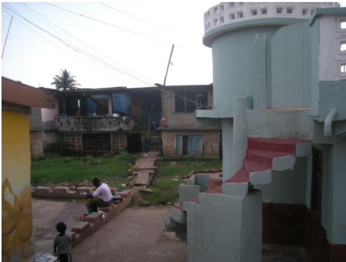
Fig. 9 Adaptation to flood by raised walls and raised wooden walkways between two houses in Kumasi
