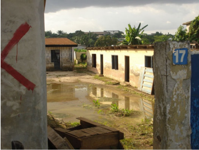
Fig. 12 A house marked for demolition by the KMA in a flood-prone suburb of Kumasi
