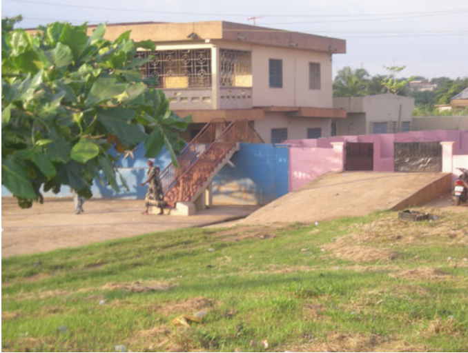
Fig. 10 Adaptation to floods by building a wall around house. Note the raised car ramp and staircase into the house
