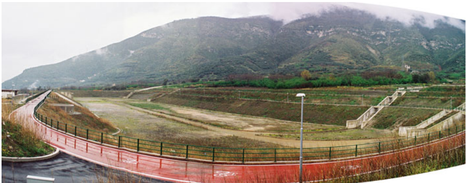
Fig. 9 Debris basin at Sarno in Italy. A cycle track has been incorporated into the perimeter of this feature as an amenity for the local population. (This picture is a photo-collage and some distortion is inevitable)
