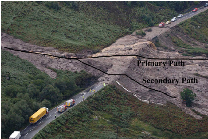
Fig. 3 Debris flow at Glen Ogle on the A85 road in Scotland, UK. This was one of two debris flows that blocked the road on 18 August 2004. Some 20 vehicles were trapped between the two flows, and the 57 occupants were airlifted to safety by helicopter and the road was closed for 4 days. The photograph shows the primary path of the debris as it passed first, and briefly, through a culvert and then overtopped the road and the secondary path as a rock outcrop was overtopped sweeping one vehicle away as illustrated in Fig. 4
