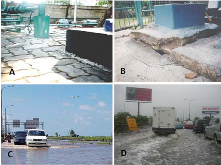
Fig. 14 Several indication and impact of land subsidence in Jakarta (Wirakusumah 2008). a and b are locations in Kamal Muara; c and d are locations along the highway to the airport (Cengkareng)
